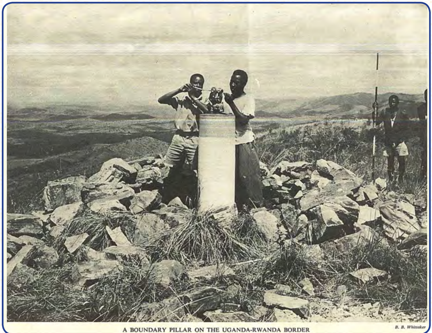
Figure 7: An international boundary pillar.
